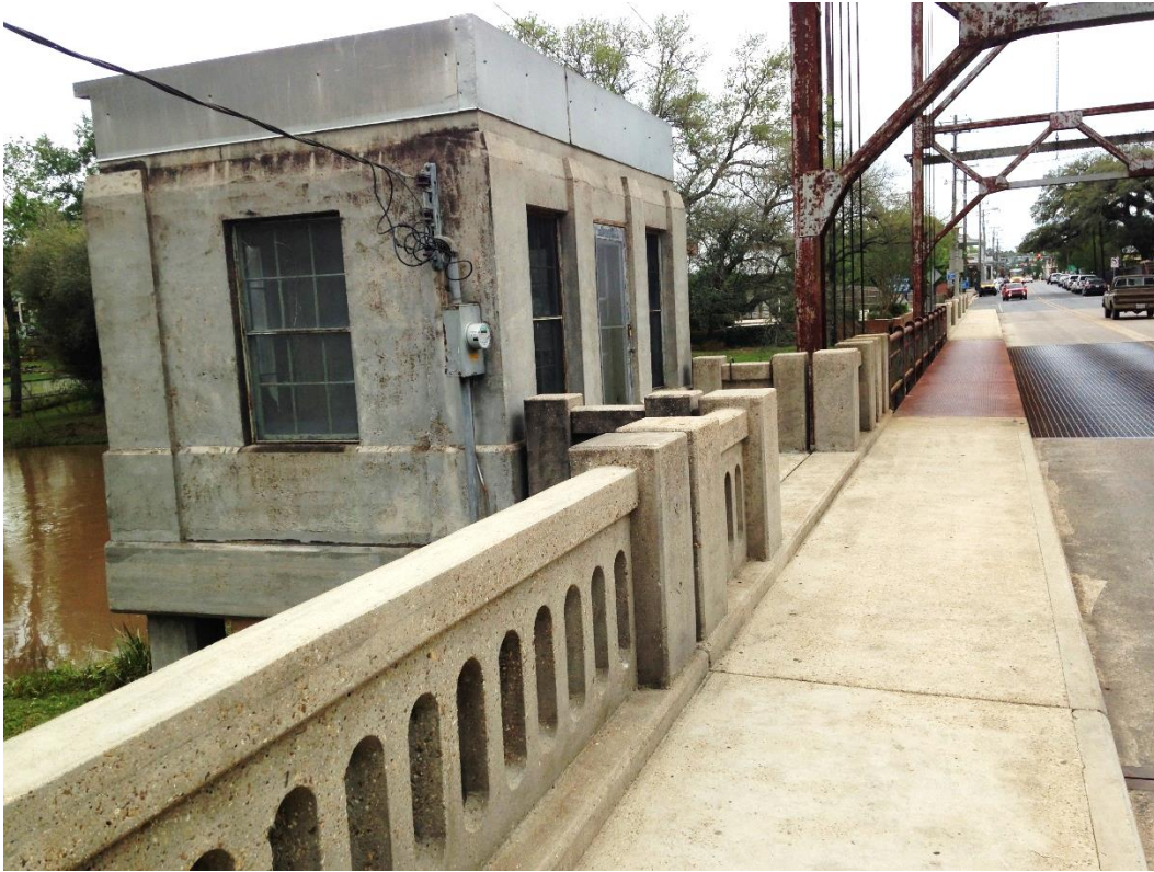
Historic Fabric Photo 3: Bridge operator's house.
