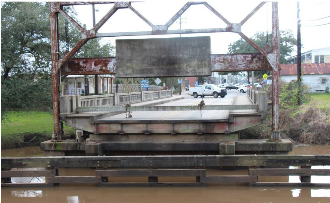
Condition Photo 12: Lift span partially open; condition of bridge components.
