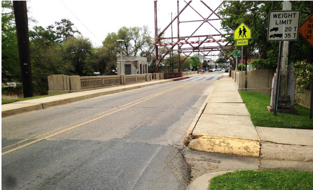
Condition Photo 4: East approach spans concrete deck, sidewalk, concrete railing.
