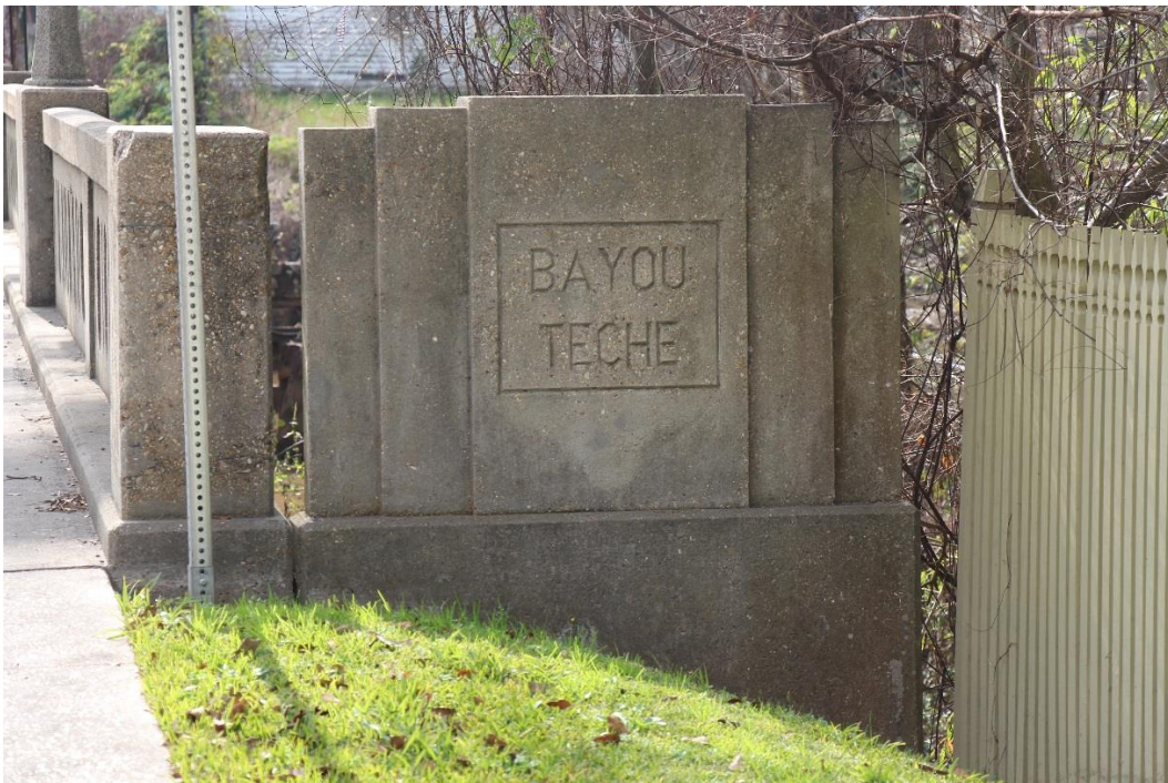
Historic Fabric Photo 2: Endposts on decorative concrete railing of approach spans.
