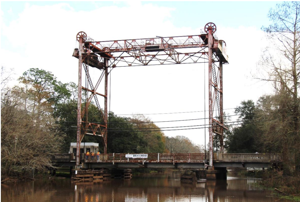
Character-defining Feature Photo 1: Design and construction of a vertical lift span with central drive machinery. The operating machinery, located at the center of a platform, drives the four sheaves on each corner of the lift towers.
