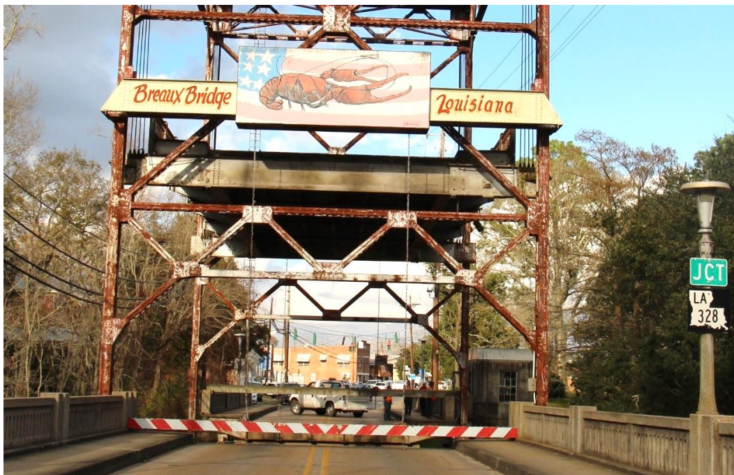
Condition Photo 13: Bridge up; traffic barrier gate, counterweight, general bridge condition.
