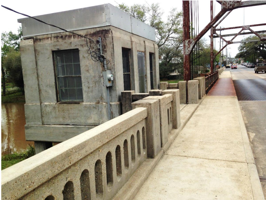
Condition Photo 18: Operator's house exterior condition.
